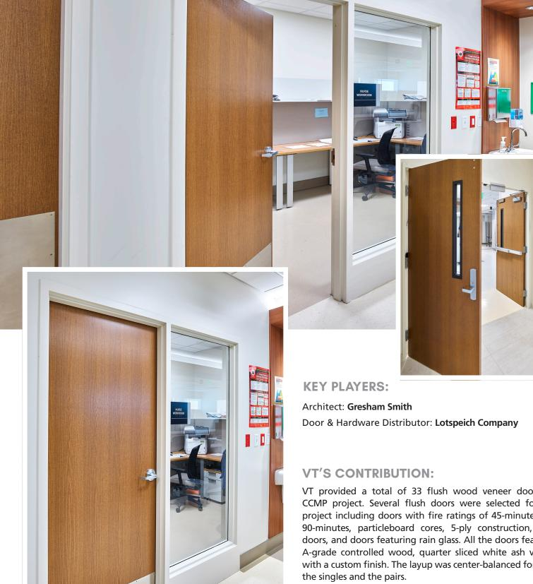
VT provided a total of 33 flush wood veneer doors for CCMP project. Several flush doors were selected for this project including doors with fire ratings of 45-minutes and 90-minutes, particleboard cores, 5-ply construction, barn doors, and doors featuring rain glass. All the doors featured A-grade controlled wood, quarter sliced white ash veneer with a custom finish. The layup was center-balanced for both
