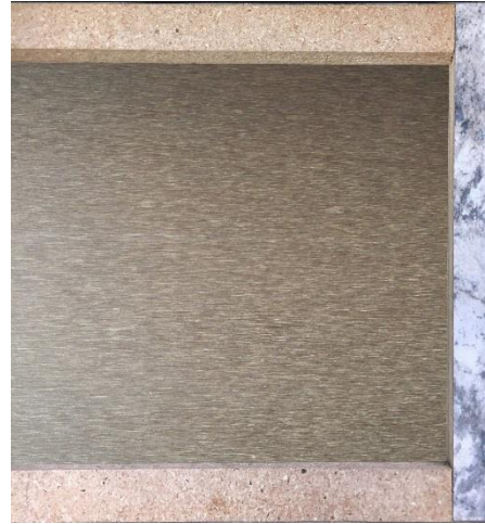
Underside of a laminate countertop with backer
