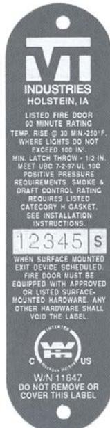
It also includes required building code information for the intended use of the door, such as maximum temperature rating. (Note: The smoke or "S" rating is achieved only after surface applying an approved smoke gasket around the perimeter of the frame.)<sup>8</sup>
